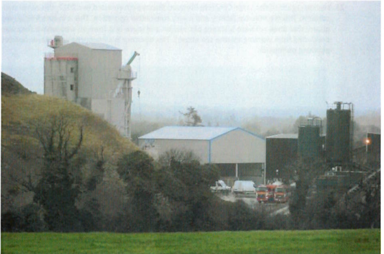
Construction of plant in 2016 without planning consent
